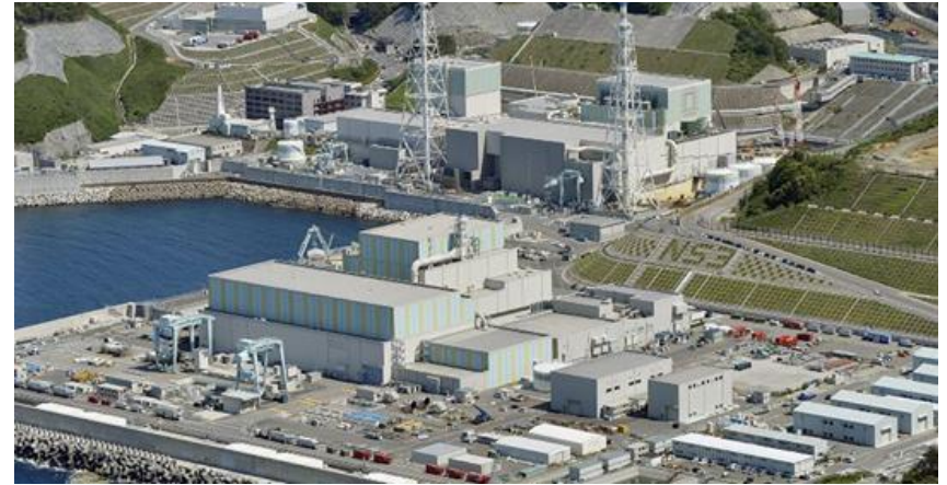
Shinjoh 1&2, with Shinjoh under construction 3 in foreground (Kyodo)
