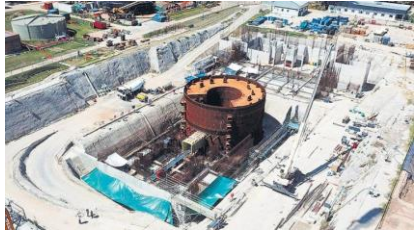
Carem 25, Argentina 25 MWe PWR Under Construction
