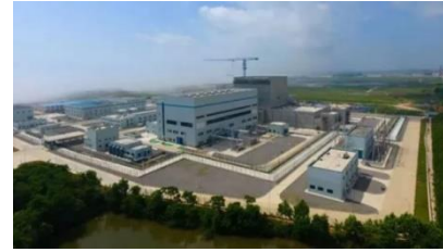
HTR-PM, China 2x110 MWe HTGR Under Commissioning
